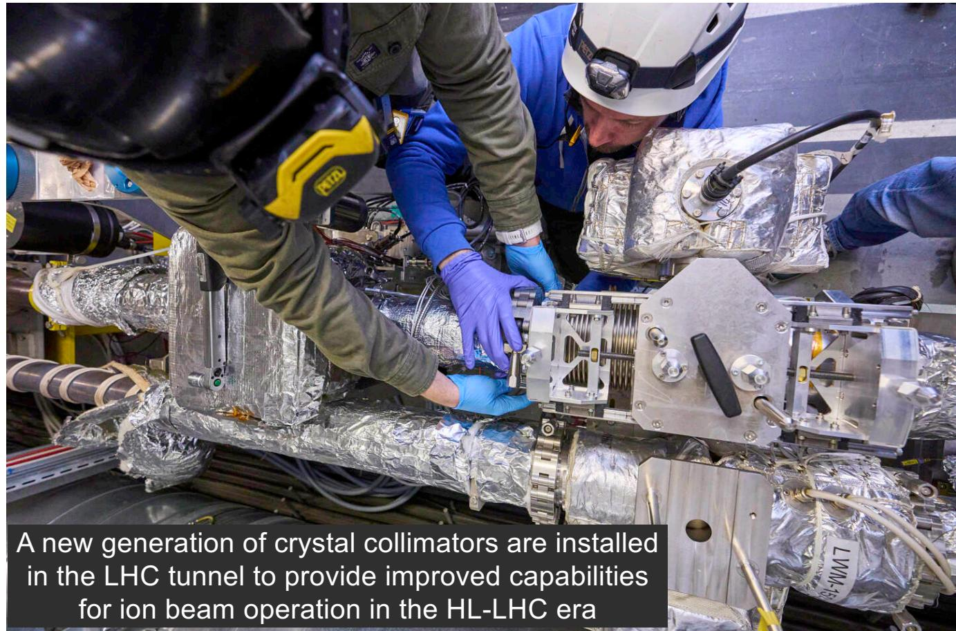
A new generation of crystal collimators are installed in the LHC tunnel to provide improved capabilities for ion beam operation in the HL-LHC era
